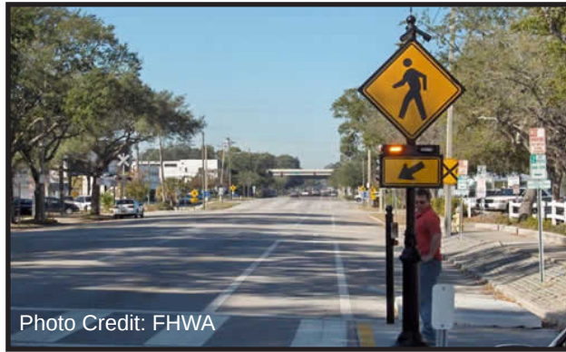
Figure 21 - Rapid Flashing Beacon
