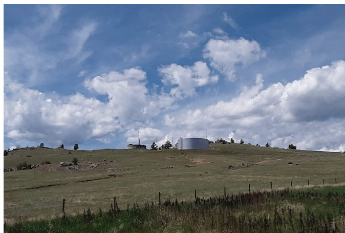
Storage Tank Facilities
