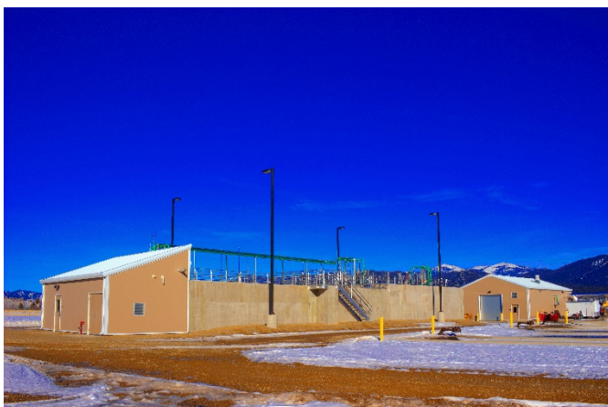
Wastewater Treatment Facility
