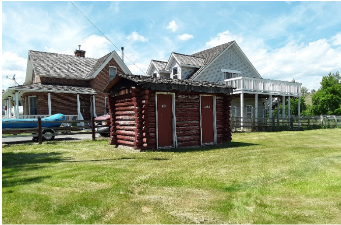
Eastside Park Restroom
