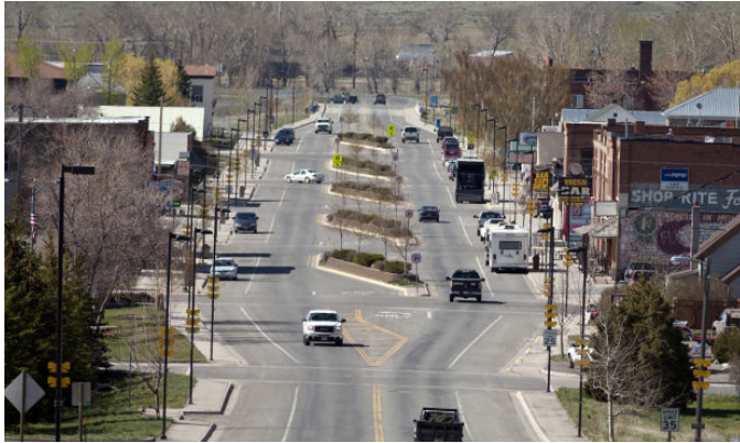
Main Street, Boulder Montana (Photo Courtesy of the Missoulian)
